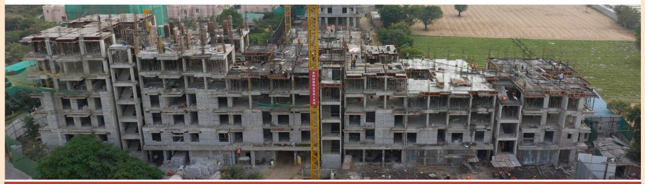
TOWER 6 - LAYING OF SECOND FLOOR ROOF TOWER 7 - LAYING OF FOURTH FLOOR ROOF TOWER 8 - LAYING OF FOURTH FLOOR ROOF
